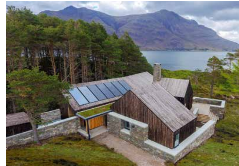
Above: SIPs provided the ideal build method for this home, as the owner wanted to create a low-energy house in this stunning off-grid location. JML SIPs designed, manufactured and erected the SIPs kit. Below: This project, by SIPs@Clays, shows the construction process on site
